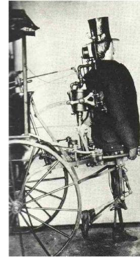
Figure 1.1: In 1868, a “Steam Man” was patented. Its torso was the boiler and its body was mounted upright onto a carriage. Using legs it could walk and steer while pulling a load in the carriage. It is rumored that US President Ulysses Grant once rode in the carriage, called the “Devil’s Car”.
